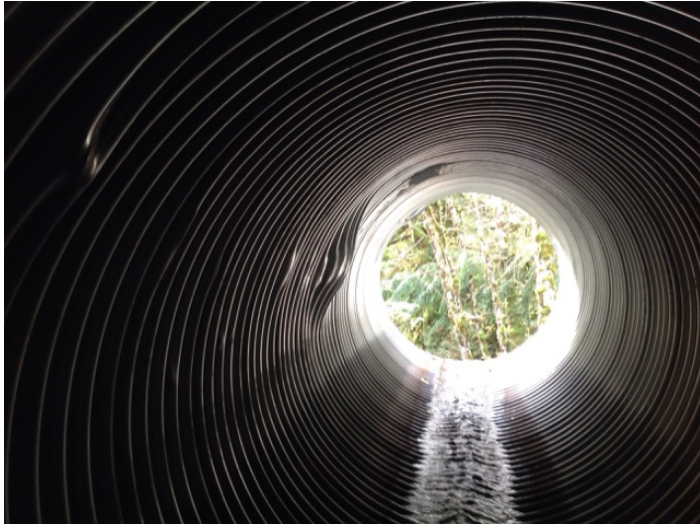
sidewall damage
