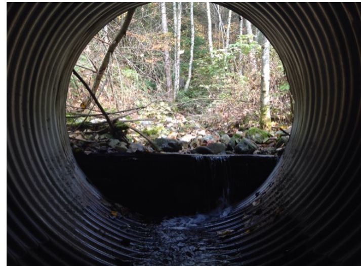
Inlet partially obstructed
